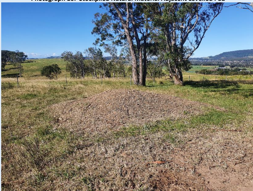
Photograph 16: Stockpiled Natural Material Adjacent Levelled Pad
